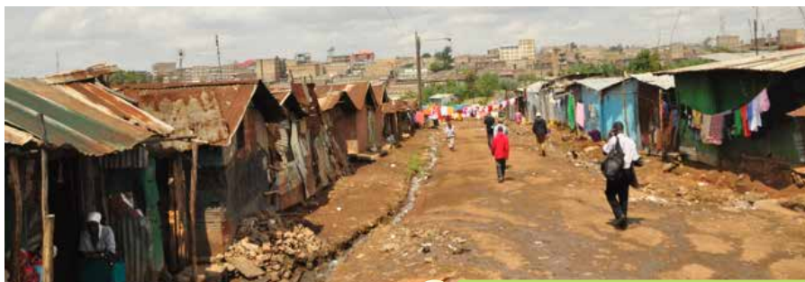
1 This is Korogocho slum in Nairobi where the PAMANECH project under the Health Challenges System (HCS) program is being implemented. Estimates show that 58% of urban residents in Kenya live in urban informal settlements, also known as slums.
