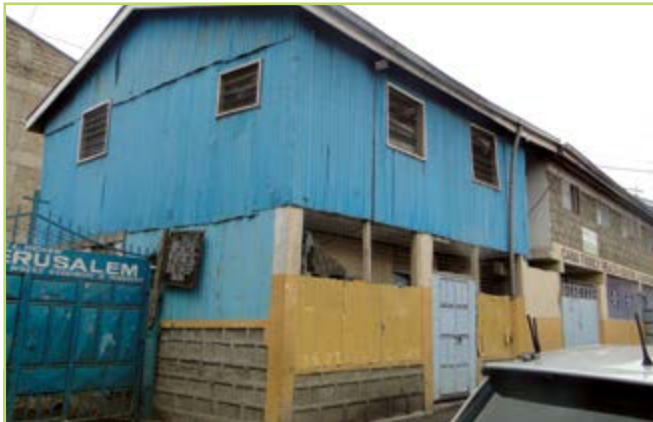
Cana Health Facility Before Construction
